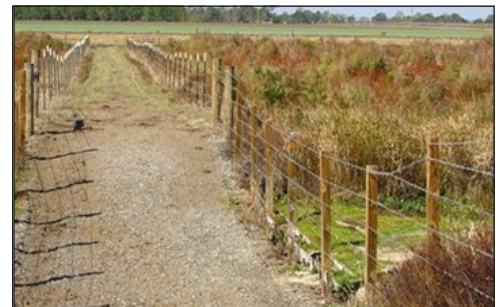
Fencing restricts livestock access to the crossing
