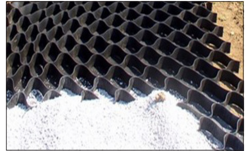
Cellular confinement panels being backfilled with gravel
