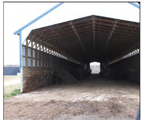
Protection around a waste facility.
