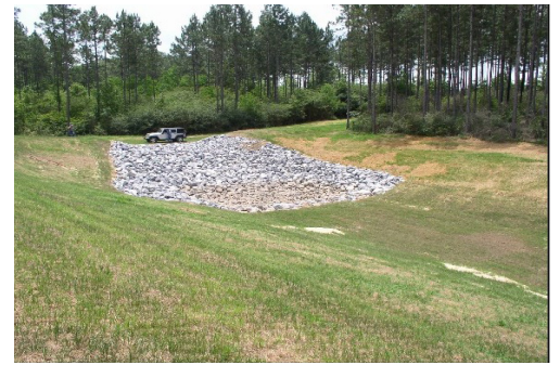
Rock Chute at end of waterway.
