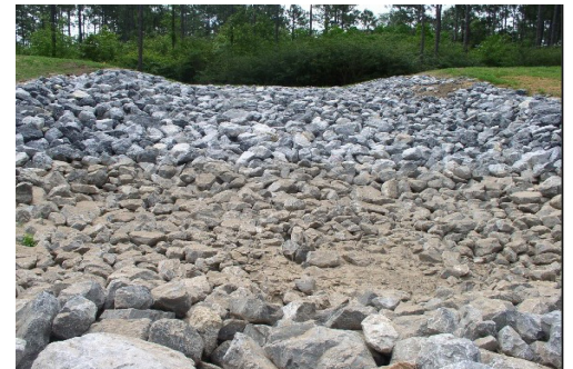
Proper rock size is critical for success of structure.
