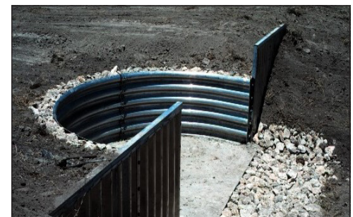
Grade stabilization structures can combine different materials.
